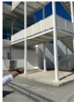
Figure 8 Showing Gate 7 Emergency Exit
