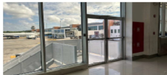
Figure 7 Rotunda Emergency Exit - Inside
