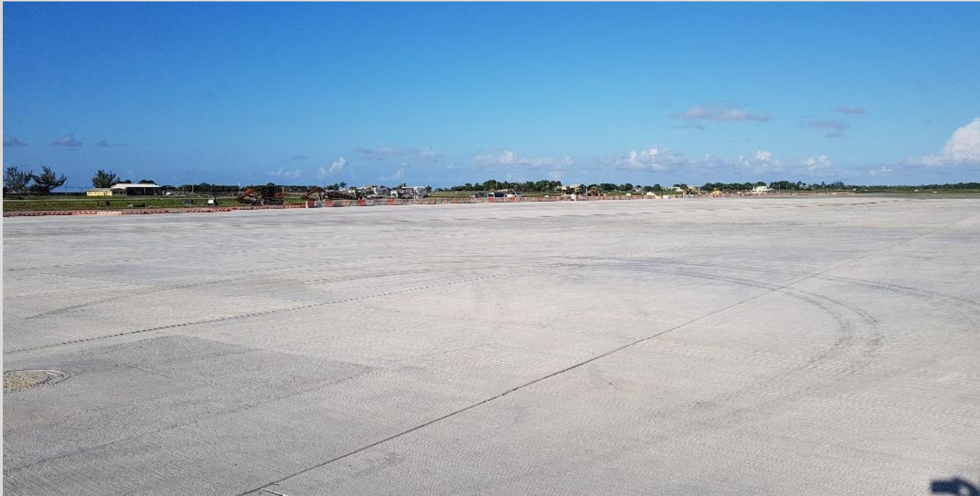
Rehabilitated Taxiway Foxtrot (Previously Asphalt, now PCC)
