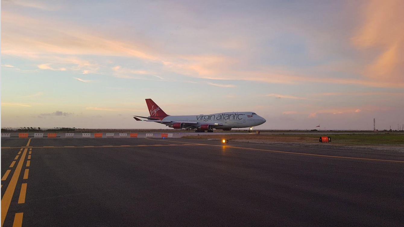
Rehabilitated Taxiway Alpha between RWY 07 and TWY D
